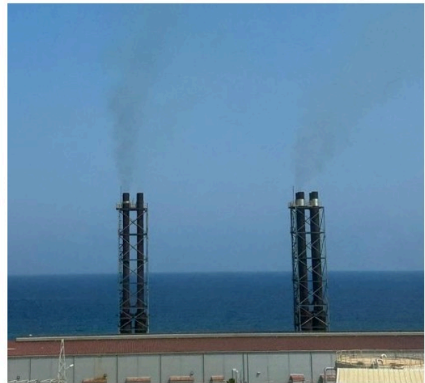
Figure 20 Diesel Generator Chimneys
