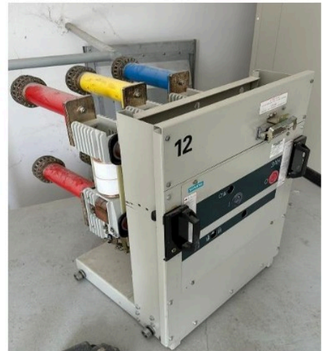
Figure 25 Circuit Breaker with vacuum inside
