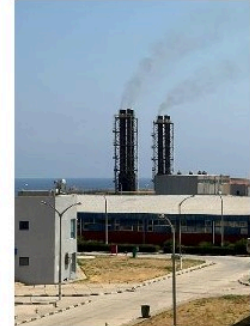
Figure 17 Diesel Generator Chimneys (8 Chimneys for 8 Generators)
